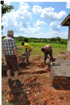
started by laying the bricks for the platform that they water tank will sit on. They crushed some of the bricks to fill in the base and then poured the cement on top. Inside the health centre they started to install the pipes for the system as well. David, Iain, and Ted
